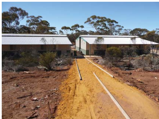
Figure 5: Installation of concrete paths for new camp.
