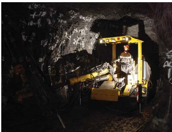
Figure 2: Ring drilling for stoping production.
