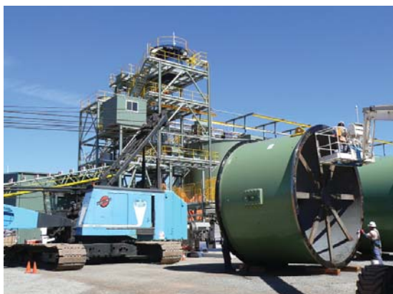
Figure 3: Delivery of ball mill shells to site.
