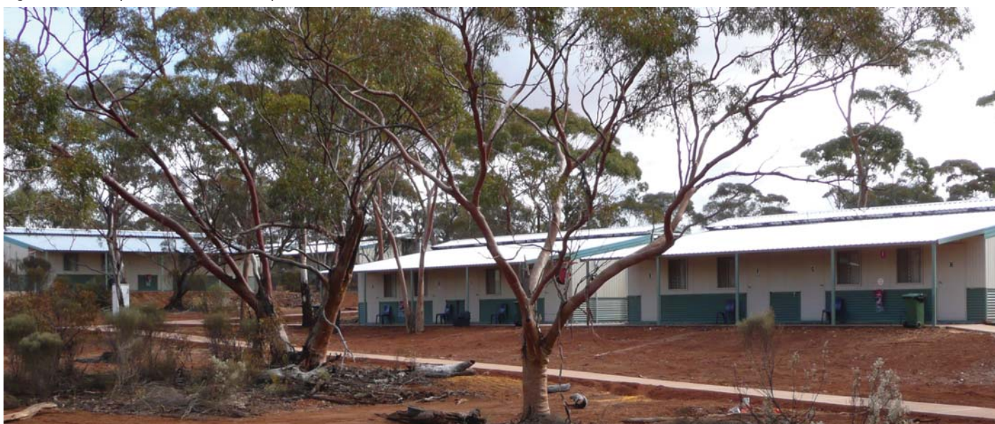
Figure 3: New camp accommodation is complete.
